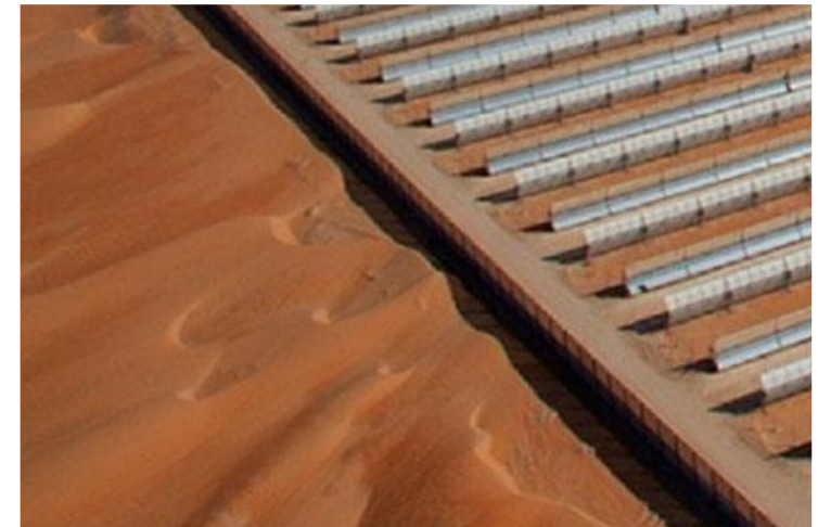
Shams 7 m high Wind Break Barriers
