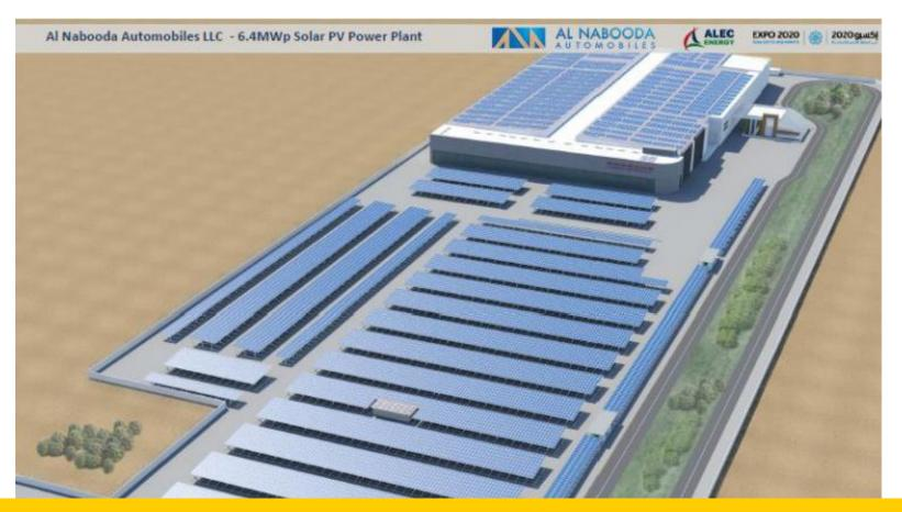
Over 25,000 solar panels will be installed at Al Nabooda Automobiles' facility. The solar plant will meet 75% of facility's energy needs and reduce CO2 emissions by 6,000 tons.
